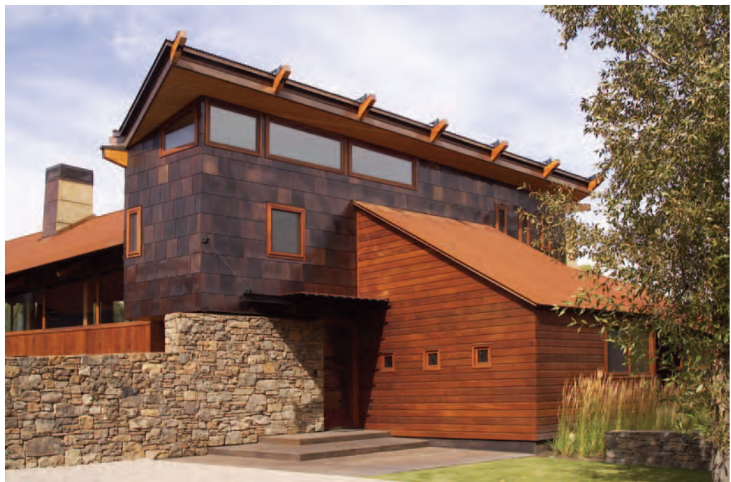
Residence 3, Exterior: Entrance with copper shingles, rusted steel roof, stone wall and wood siding.
