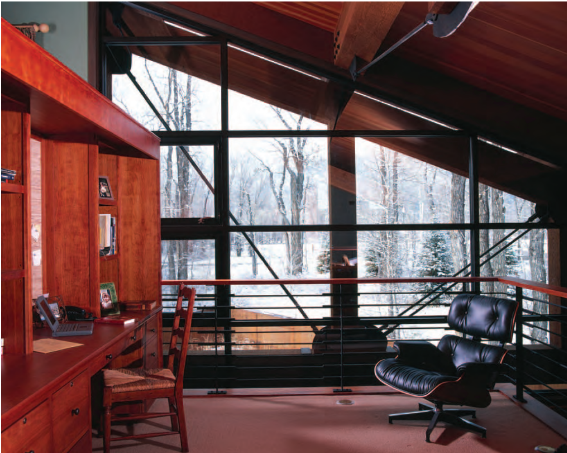
Residence Interior view: The timber truss permits uninterrupted glass wall and sun shading.
