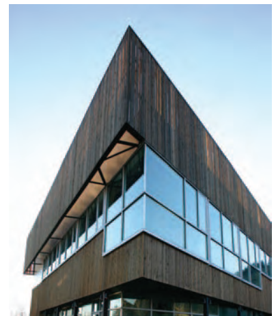
Commercial Building: Light filters through the wood slatted sun shading and mechanical equipment screen.
